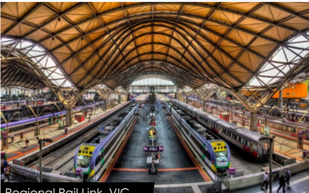
Regional Rail Link, VIC
