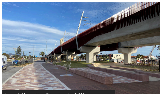
Level Crossing Removals, VIC
