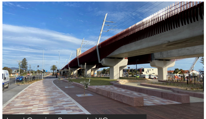
Level Crossing Removals, VIC
