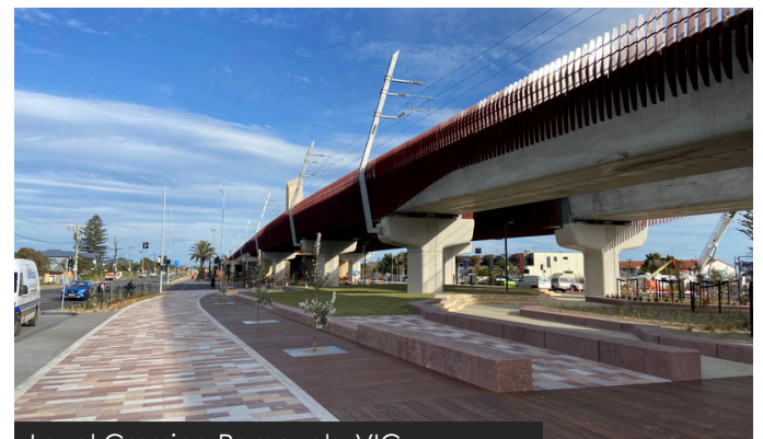
Level Crossing Removals, VIC
