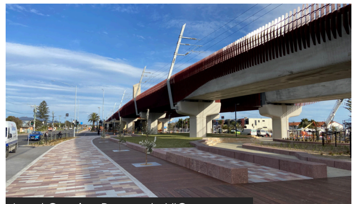
Level Crossing Removals, VIC
